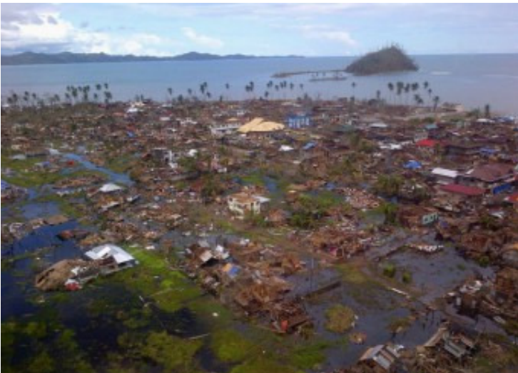
Aerial view of damaged houses.
